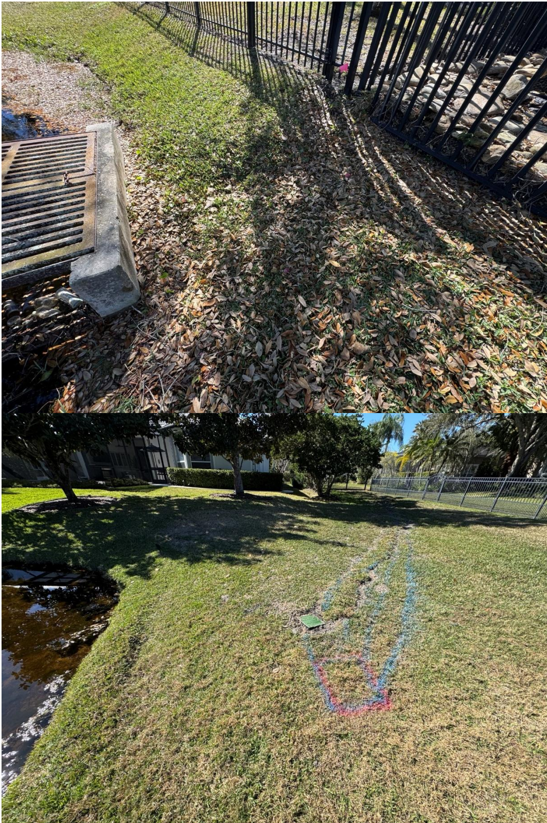
Photo 6 – Displays Pond 9 control structure with minor erosion on the back side of the structure and the french drain installed on CDD property at the NW corner of the pond. The french drain appeared to be coming from 12046 Royce Waterford Cir
